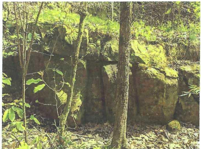
Shades Mountain Cut drill marks. Birgit Kibelka, 2017.
