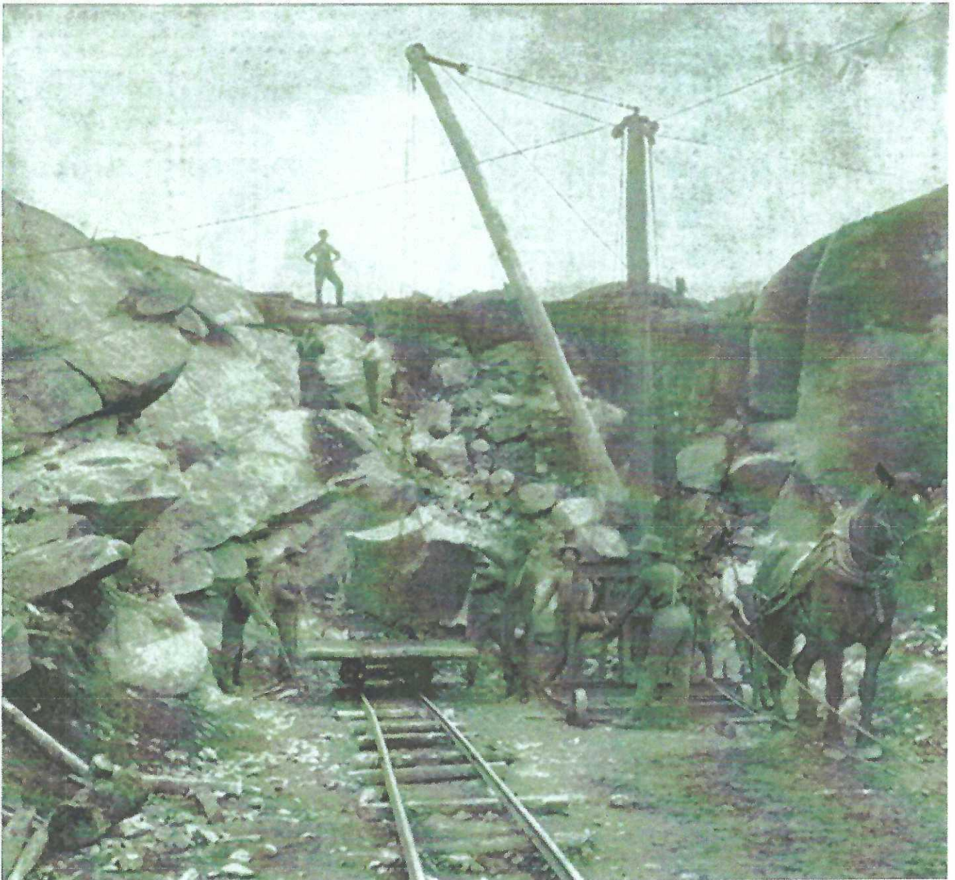
Working in a rock cut at Smithville, Minnesota, using a steam-powered derrick, similar to that used at Brock's Gap, to lift and haul massive stone following a blast. National Iron Company, Engineers and Designers of Steel Structures ad. Courtesy Bob Yuill.
